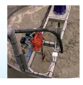
The screw separator (A), or the dewatering screen, recovers washed material.
